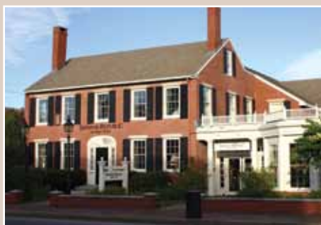
Banana Republic built a brick Federal home for its store
