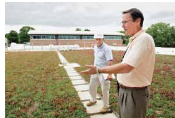
Two officials look over the green roof on Lancaster's Lafayette Elementary School.
