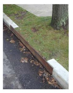
When installing new curbing, use a metal plate adjacent to the tree. Plates in various lengths are available from Pottstown Metal Welding Inc.
