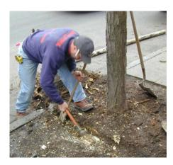
If you don't have room to go around tree roots, you can "shave" the roots with a hatchet by removing small roots and notching large ones about 3 inches below ground level to allow room for a new sidewalk over the roots.
